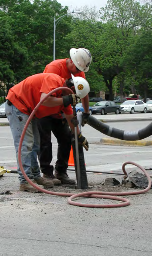
(right) Verifying the location of underground lines prior to exposing the line with vacuum excavation (above).
