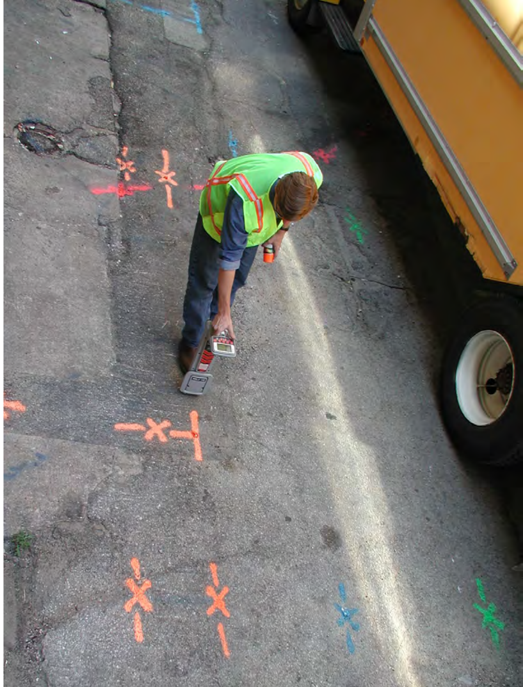
(right) Verifying the location of underground lines prior to exposing the line with vacuum excavation (above).
